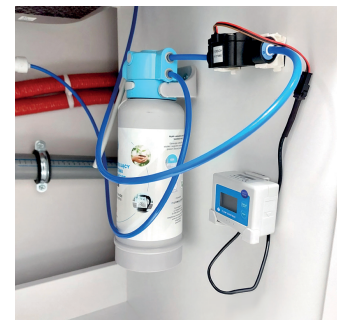
Meter installation example
