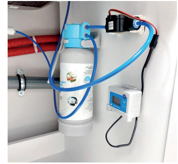
Meter installation example
